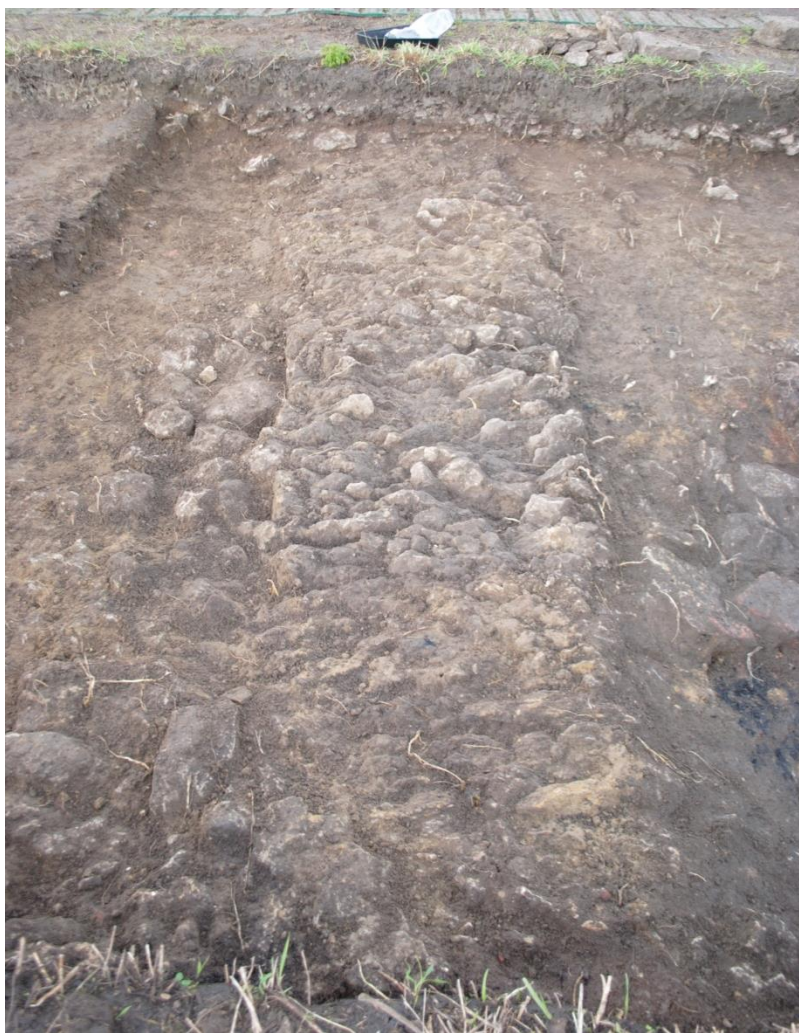
Fig. 5: looking north along wall foundation [2054], interior to right
