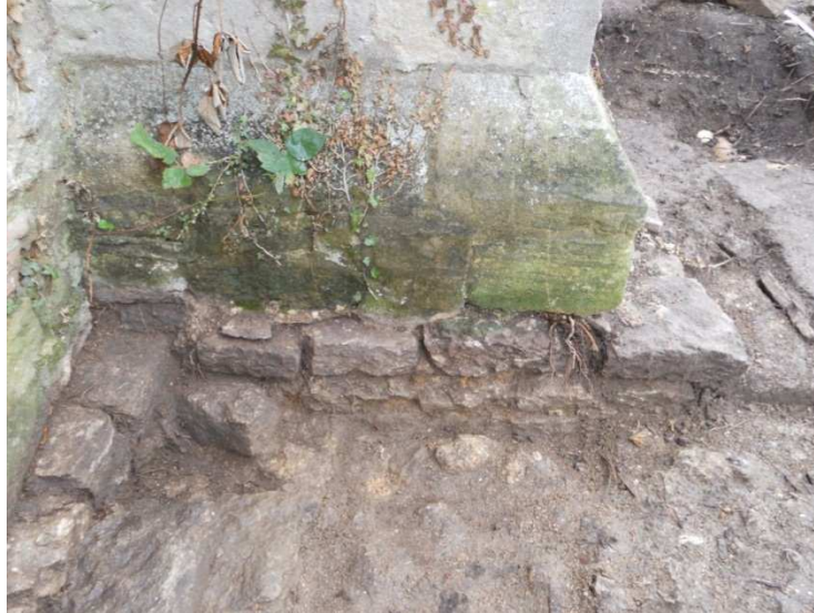
Figure 52 Central buttress: looking east
