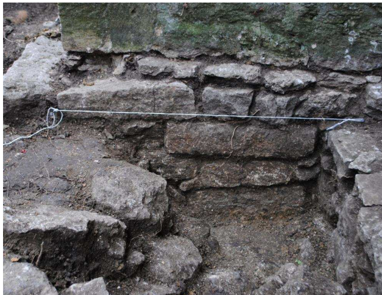
Figure 47 Central buttress: looking west
