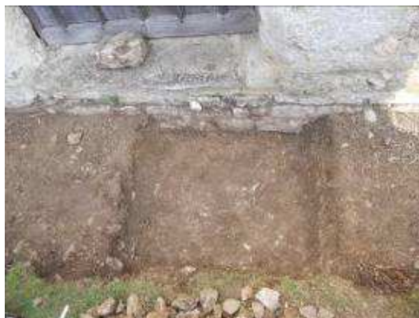
Figure 57 (1028) having been removed, the worked stone courses of masonry [1048] onto which the W elevation of the present-day chapel sits is seen to be of different stone: substantial dressed cut slabs.
