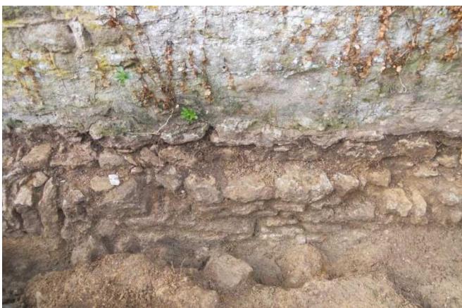
Figure 42 East wall of the Chapel with phases of rebuild: looking west
