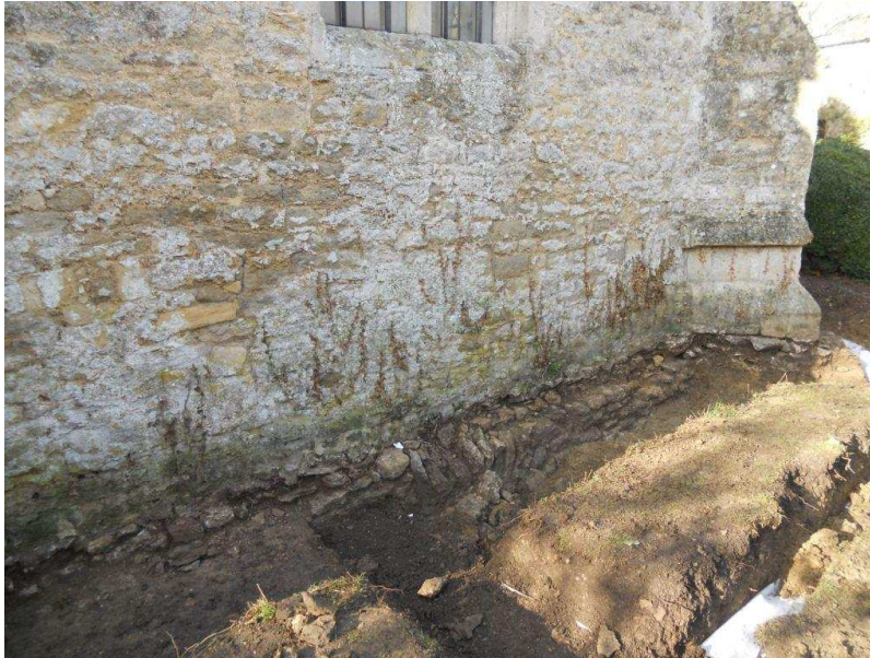
Figure 43 East wall of the Chapel: looking NW
