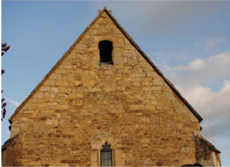
Figure 62 W gable end of chapel; the change in stonework showing clearly the raising of the chapel roof after the Civil War to give a 60 degree pitch to accommodate the hanging of a Cotswold tile roof
