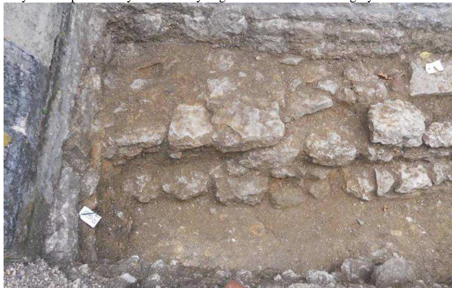
Figure 6 Eastern area of Sector A, showing the three phases of [1036] adjacent to the northern buttress. Note the area of soil below the three large flags of Phase 3 (centre left) where the upper course of Phase 2 has been lost.
