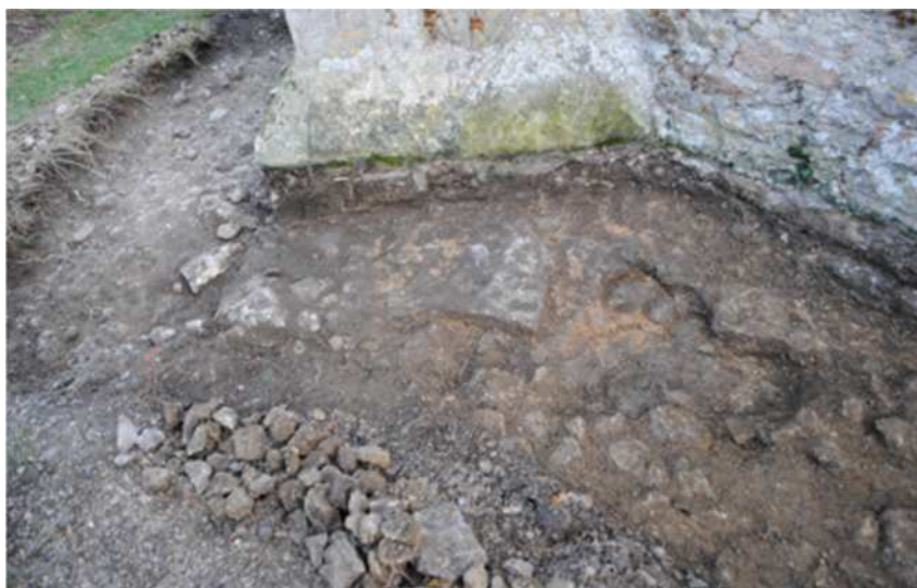
Figure 14 Eastern end of [1044] at foot of NE buttress; substantial flagstones becoming visible: south round buttress NE corner flagstones disappear: major disturbance/tumble in this area.
