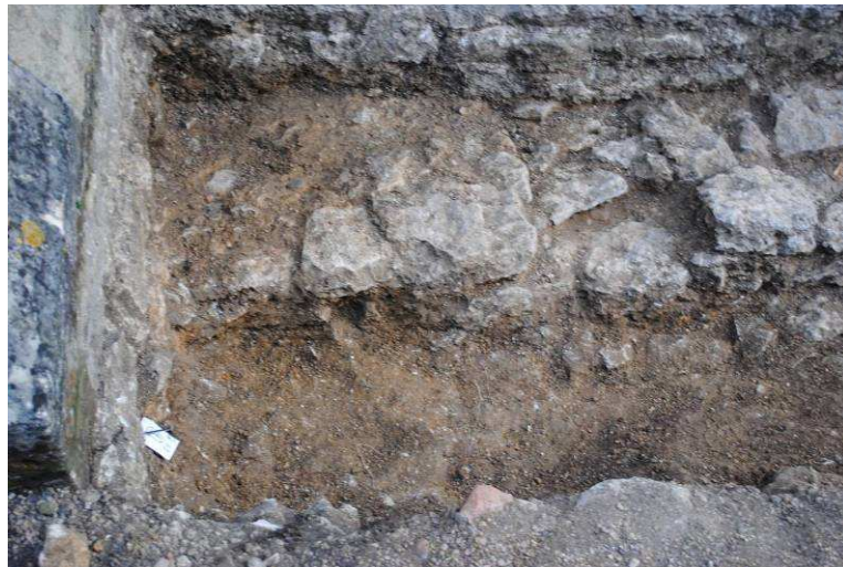
Figure 2 Showing the two patches of reddish decayed mortar (1021). The large flag at the centre belongs to the upper course of [1036], the edge of which seems to curve to the right.
