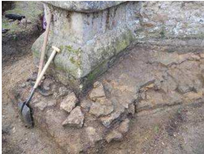
Figure 34 Flags of [1044] can be seen to NW of NE chapel buttress; the state of this structure is patchy due to disturbance/tumble particularly to the NE corner. However, the flags of [1044] can be seen to run under the NE buttress (and chapel wall at angle with buttress) and over the E end of [1037; note posthole cut/tumble in flag near angle of buttress and wall.
