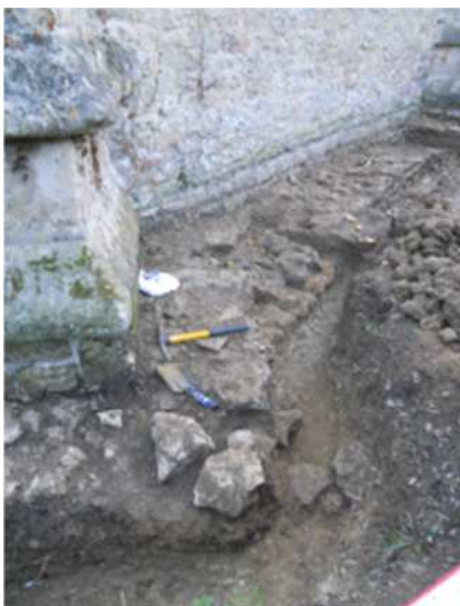
Figure 29 layer (1033) (continuing eastwards from E of (1006)), lies to N of [1037] and to S of path and continues round NE buttress and [1044] into Sector A. The wet clay base of trench to W changes to drier grittier soil rounding buttress to NE and tumble of [1044]. Note possible wall footings in trench as it rounds NE corner. Further jutting substantial lower course stones of [1037] are increasingly revealed westwards.
